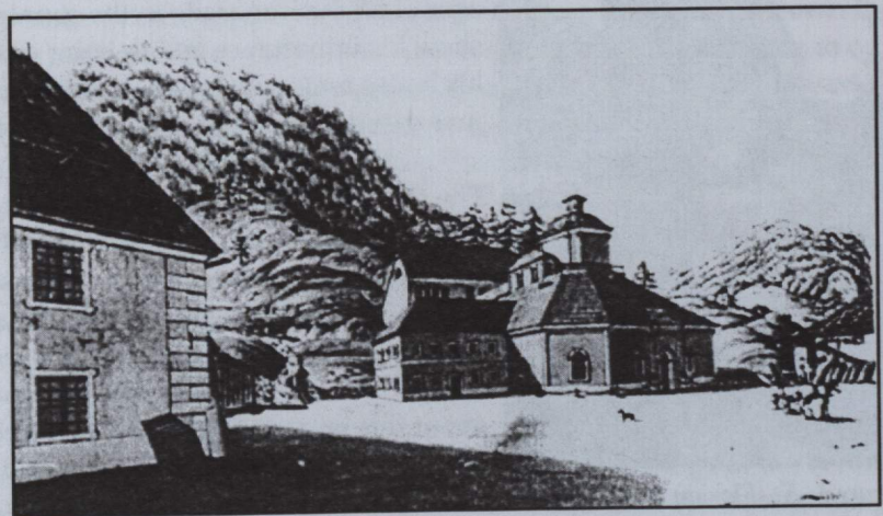
Figure 3. Furnace in Turrach, 1830.
