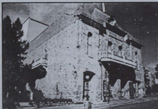
Figure 2. Central City Opera House, Colorado, 2000, showing the building’s Cornish stonework. Copyright L. Dunn.
